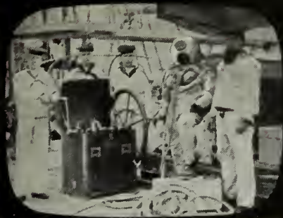
USS HARTFORD had "diving school for enlisted boys" in 1877. A hand pump on the deck supplied the air.
